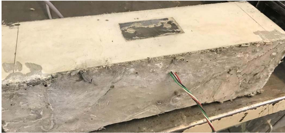
Figure 8 - Buried sensor system after concrete pouring
