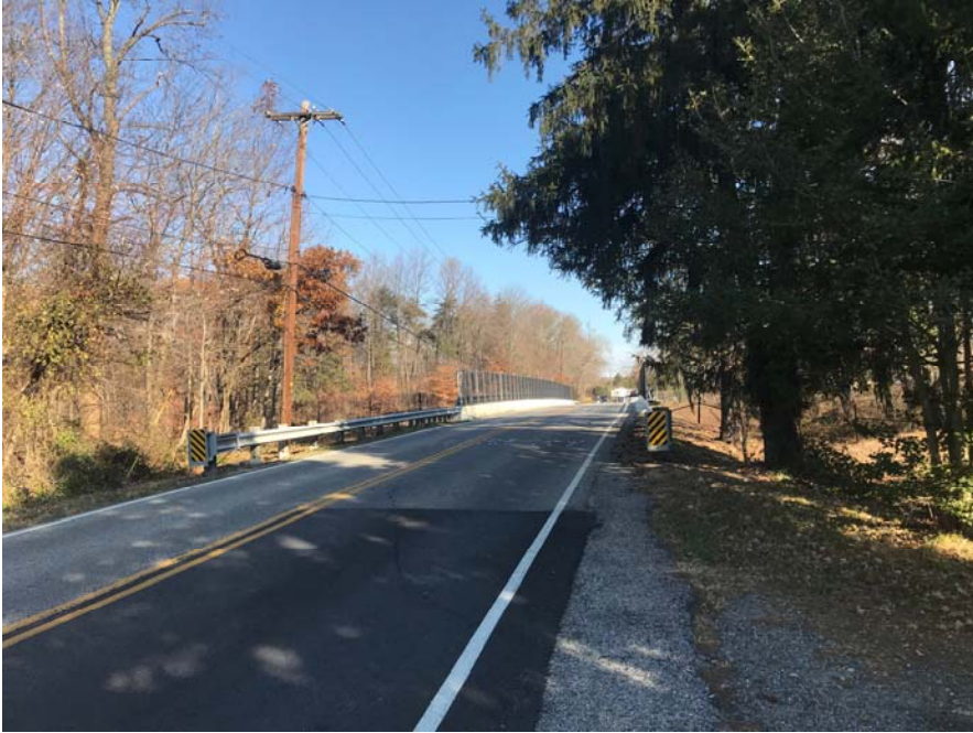
Figure A2 - Bridge CEXA27001
