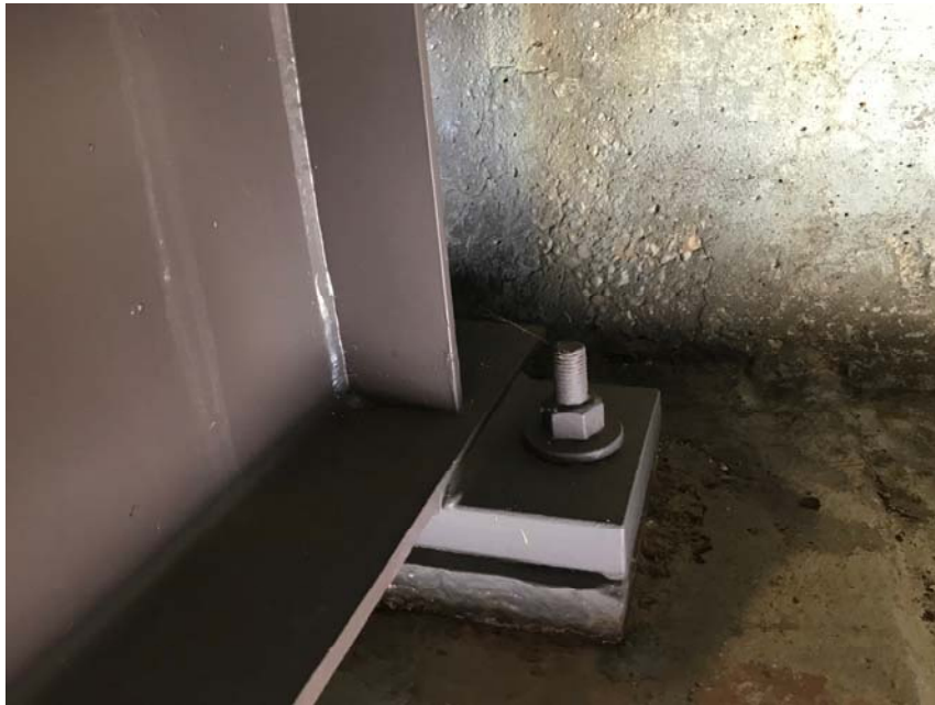
Figure A6 – Abutment fixed bearing
