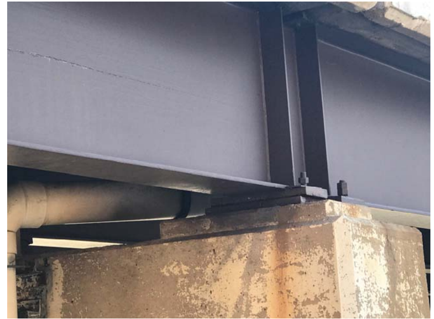
Figure A7 – Exterior pier extension bearings
