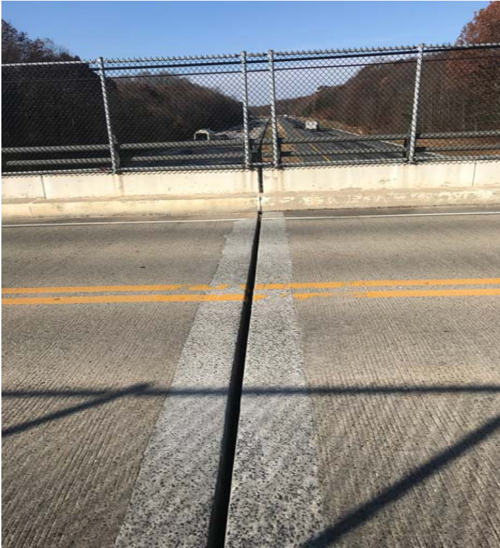
Figure A4 – Interior pier top deck expansion joint
