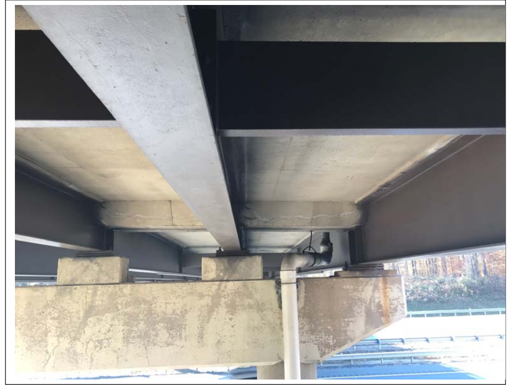
Figure A5 – Exterior pier bearings
