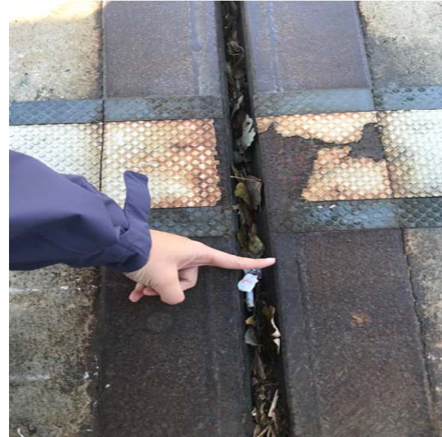
Figure A3 – Exterior pier top deck expansion joint
